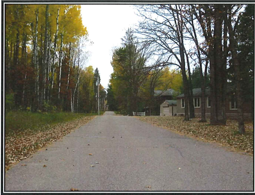
View of Existing Perkins Road
