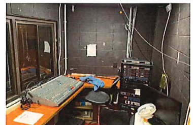
Above: Overcrowded lunch lines, ceiling leaks from worn out roofing, and obsolete auditorium technology.
