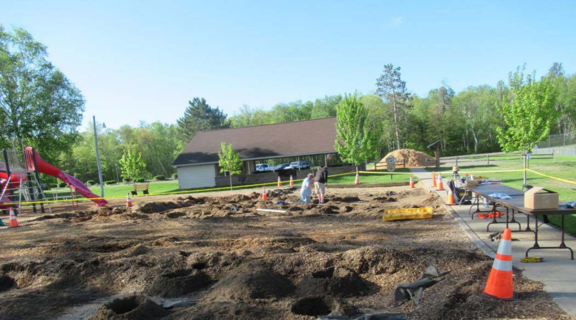
Setting the holes
