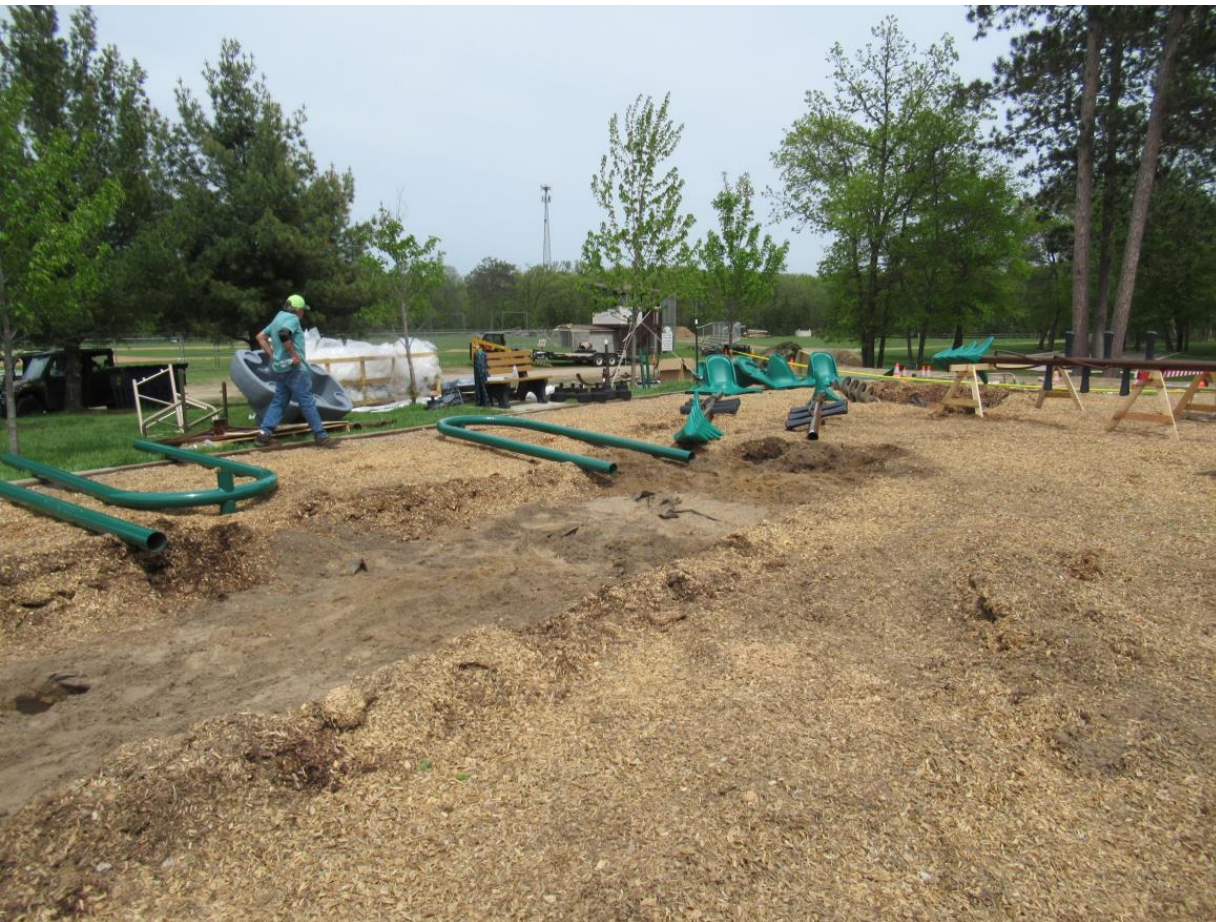
Laying out the Swing Set
