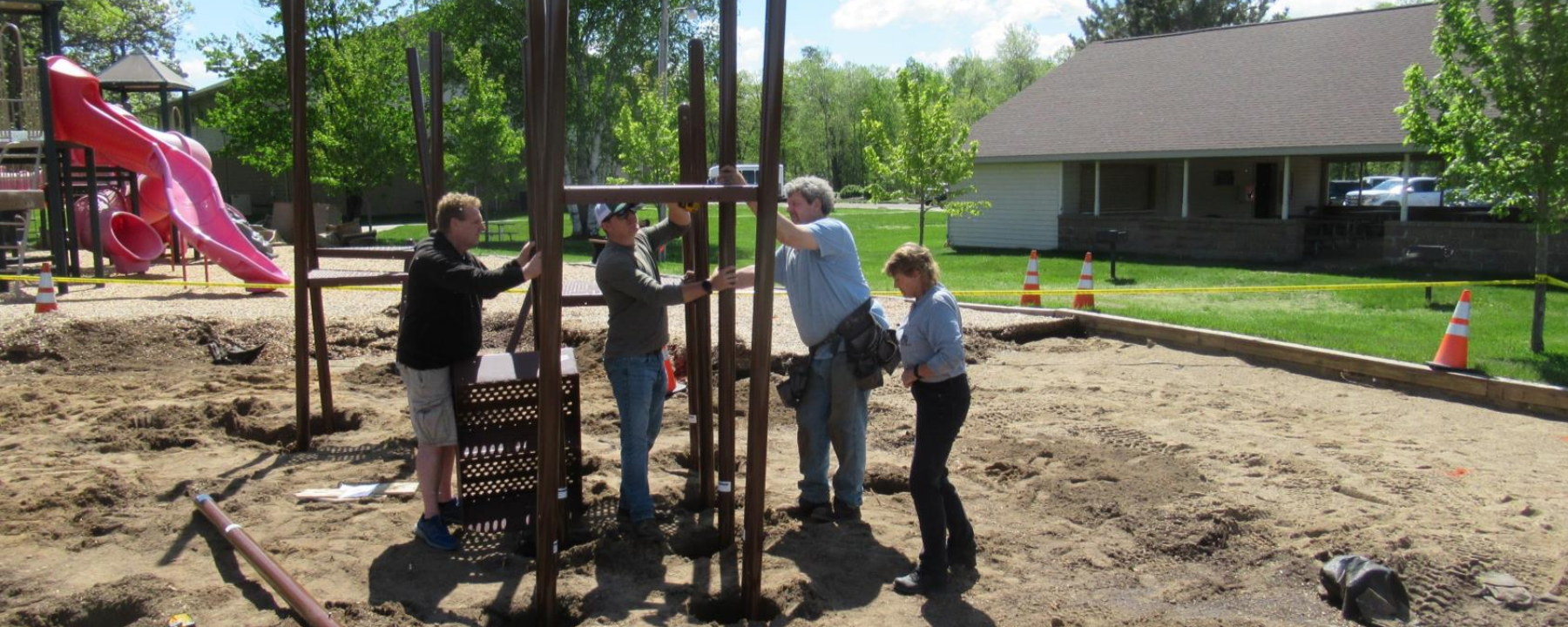
Fastening the decking to the poles
