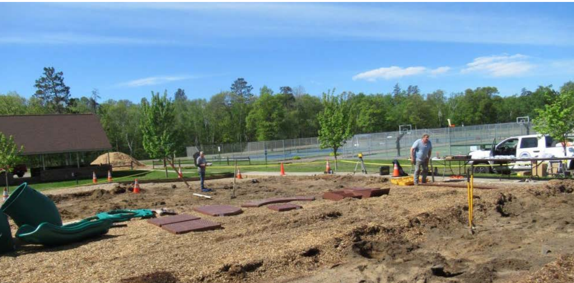
Laying out the decking
