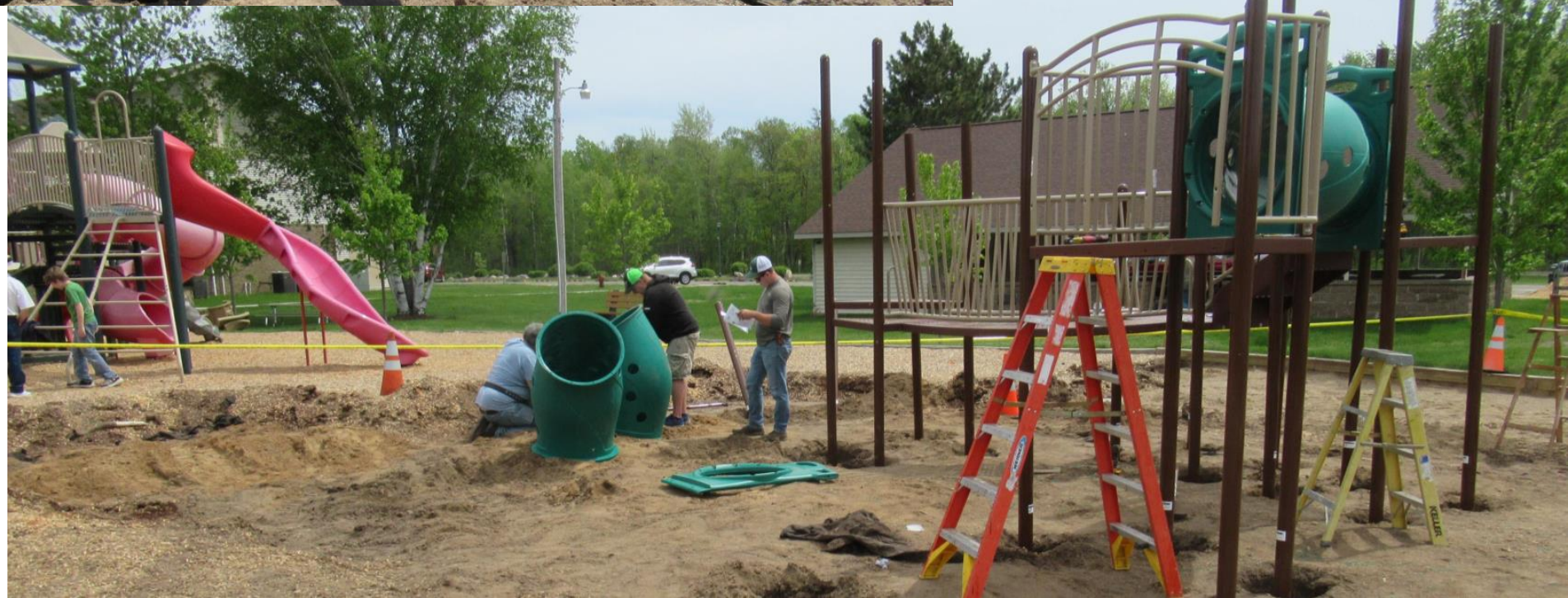
Fastening the decking to the poles
